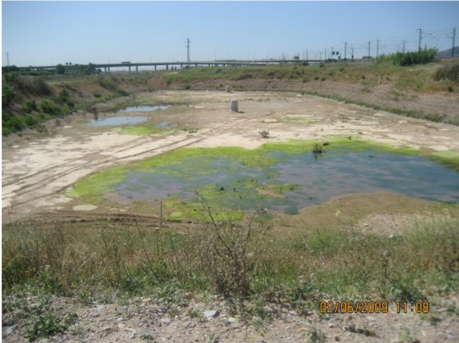
Infiltration pond after the flooding test - June 2009
